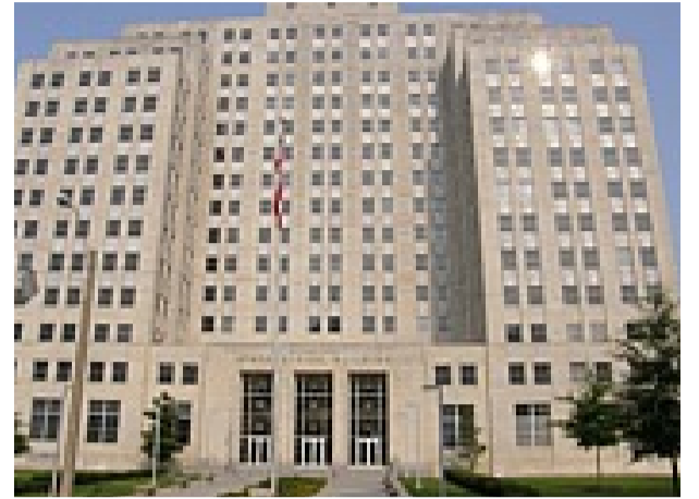
Woolfolk State Office Building
